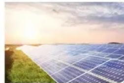
Energy Storage System
